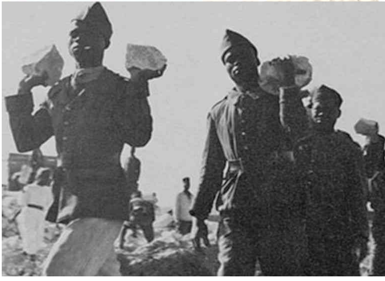
Bunker Construction, Bayonne (DR)
