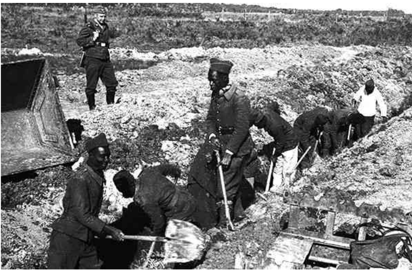
U-Bootbunker in Brest 1942 © Bundesarchiv
