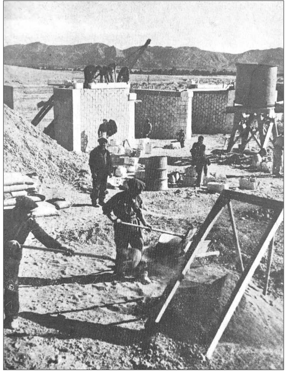
Foum Djelfa Viaduc Work, Morocco 1941 (Photo : Georges Manue)
